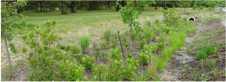
Nature-based solutions such as this bioswale capture stormwater runoff while also providing wildlife habitat.
