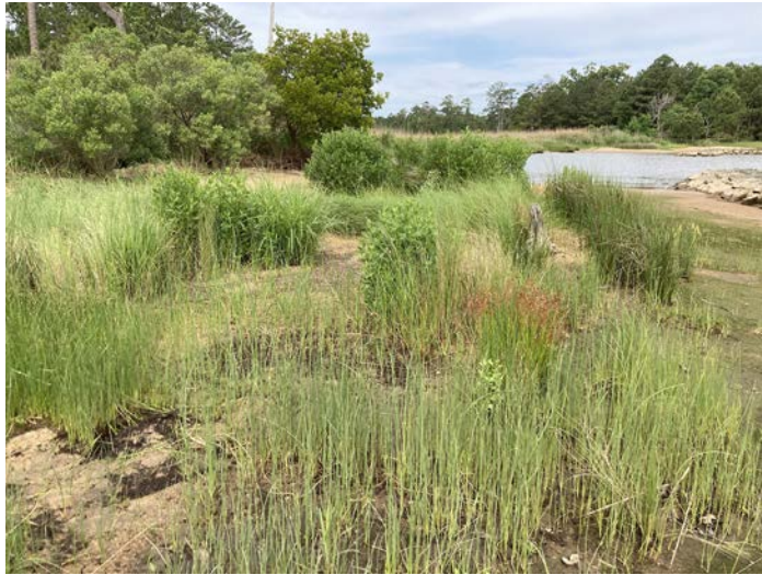
Breakers and living shorelines are being used by park staff to slowdown coastal shore erosion and keep water from penetrating further upland.
