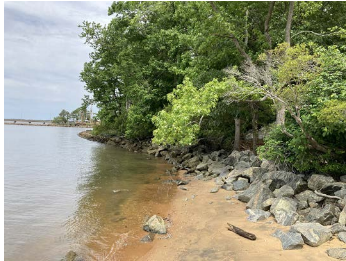
Park staff have already armored the shoreline to prevent further damage to resources, but these strategies are only effective in the short term.
