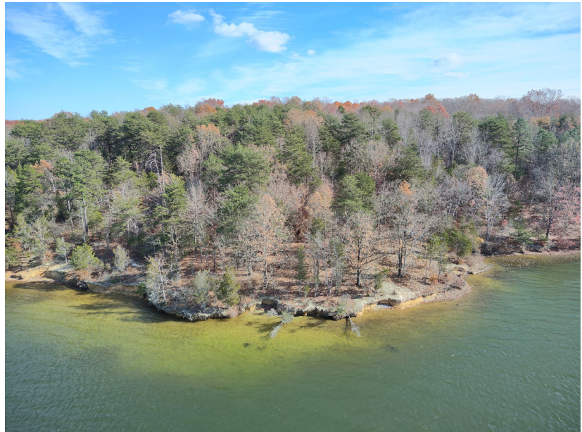
Figure 9 - Shoreline erosion at Lake Anna State Park
