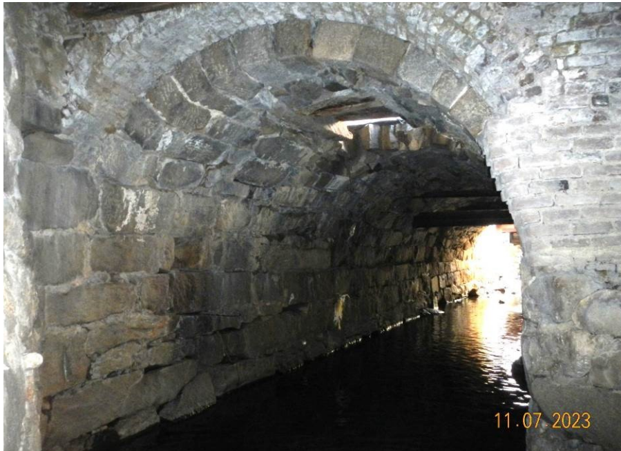
UPSTREAM (SOUTH) SIDE
